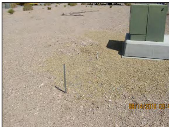
Metal pipe for electric conduit near the transformer. Gravel near transformer discolored relative to other gravel on site.
