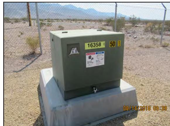
Pad mounted transformer. Valley Electric Association confirmed the transformer did not contain PCBs.
