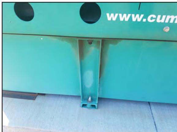
De minimis leaking on generator. Did not appear to impact soil.
